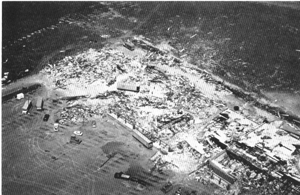
1. Remains of a shopping center in Bennettsville, South Carolina.
