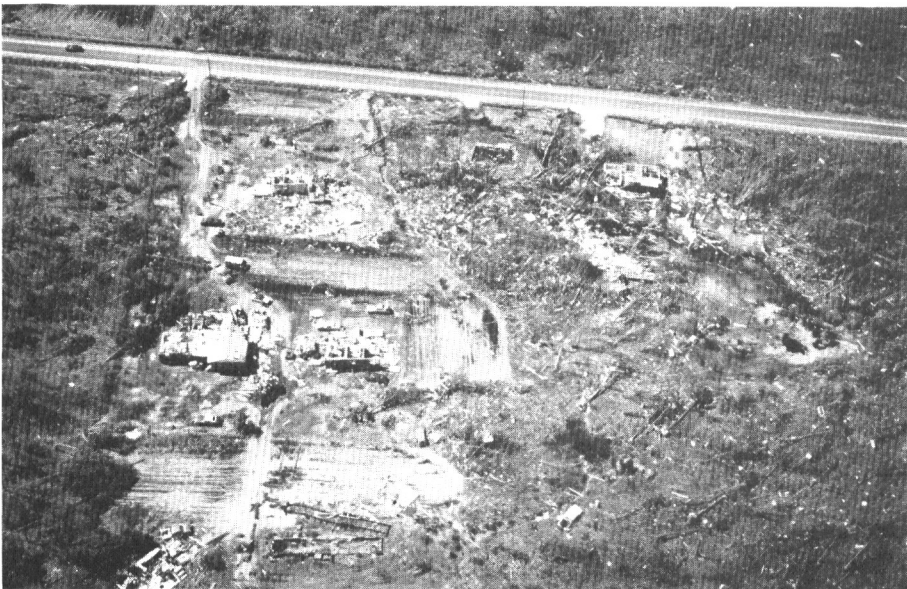
4. Total destruction of several mobile homes, and extensive damage to several frame houses SE of Fayetteville, N.C.
