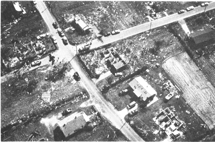
6. Selective damage to frame houses in Mt. Olive, N.C.
