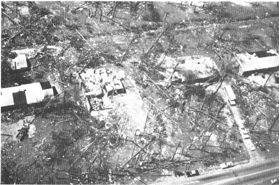
3. Selective damage in a housing development in Bennettsville, S.C.
