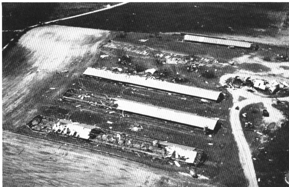
2. Damaged chicken houses near Bennettsville, S.C.
